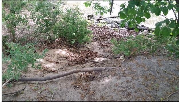
Past efforts to reduce the bank erosion by installing glacial stone has been helpful, but as seen in this picture, the soil and stone continue to slide into the lake as the bank is undercut by wave energy penetrating the voids in the stone and washing away the unprotected soil behind the stone.
