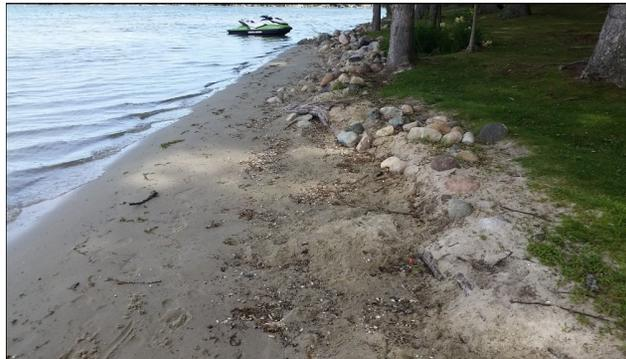
The sandy soil is eroding from behind the previously installed stone as there was not filter fabric installed under the stone to prevent erosion. The stone toe wall was not keyed into the lake bed to provide a stable foundation. The stone originally installed has slid down and is now covered with soil from the eroded bank.
